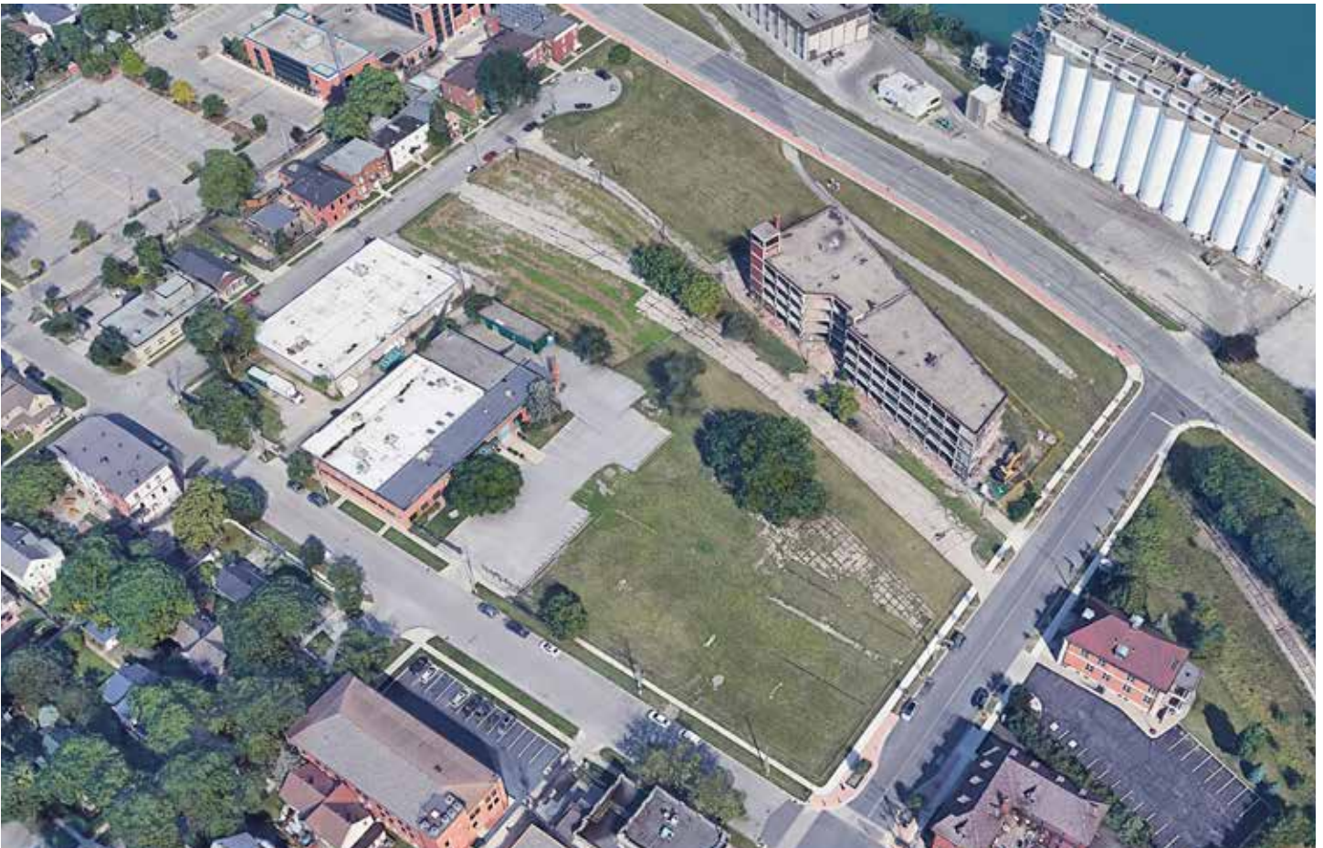
Bird's Eye View - Existing Condition
