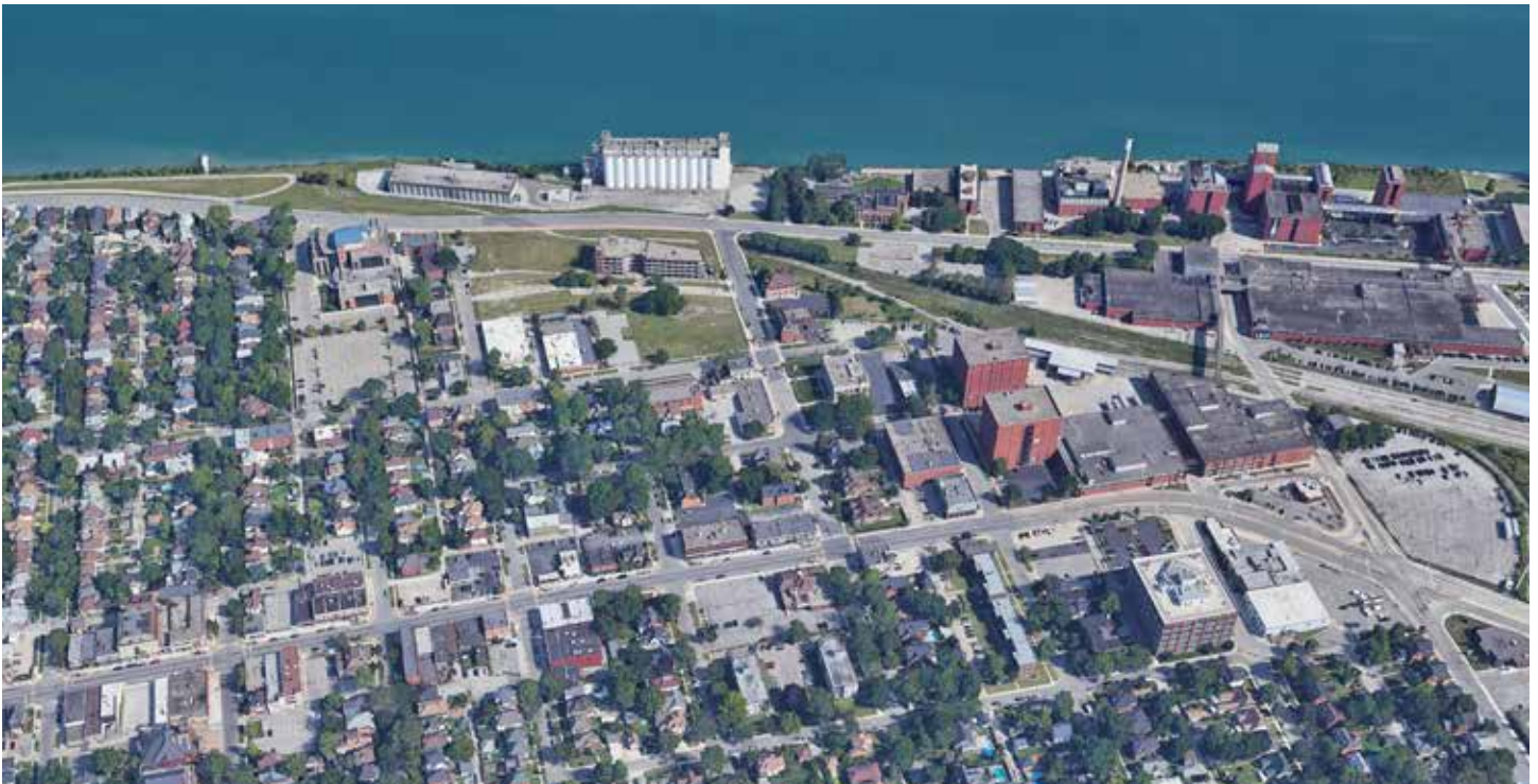
Bird's Eye View - Existing Condition
