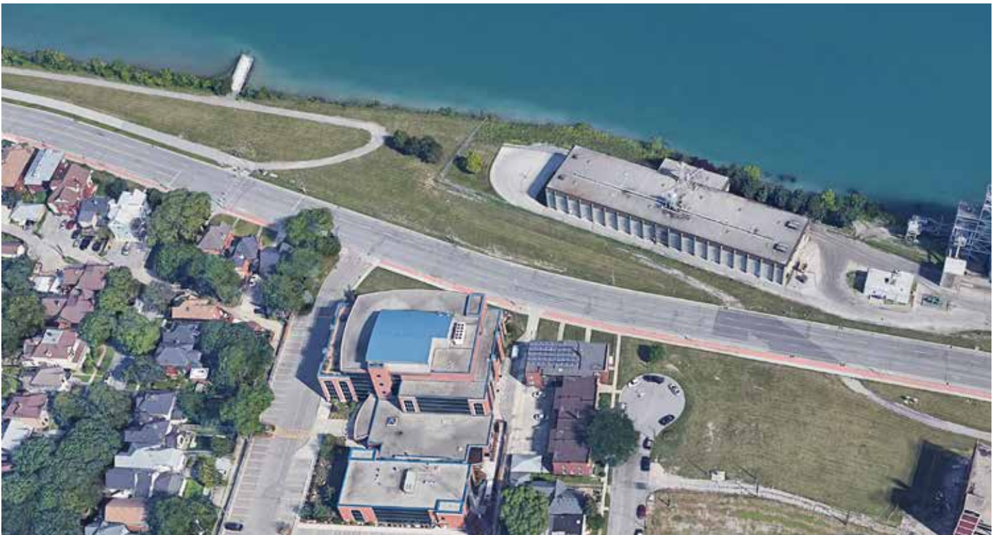
Bird's Eye View - Existing Condition
