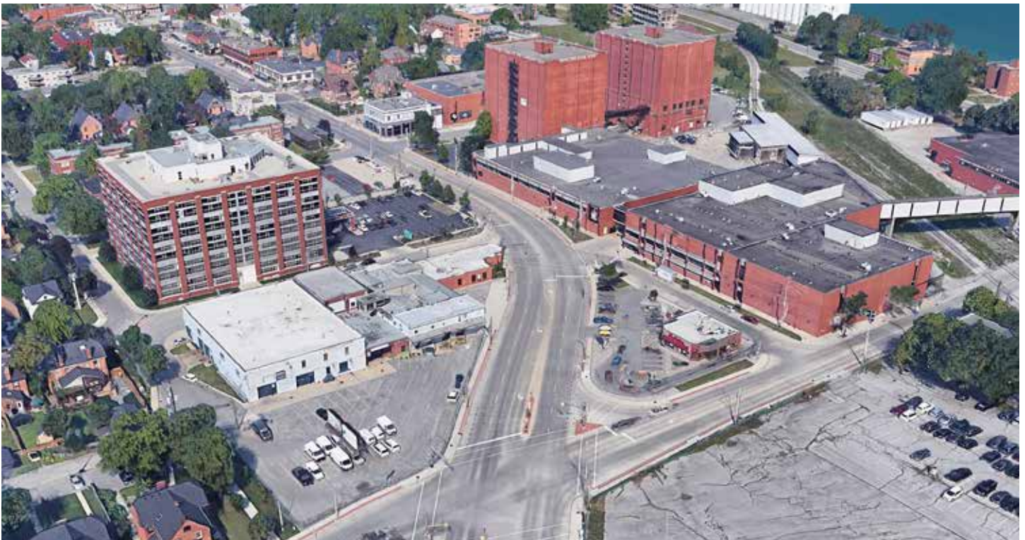
Bird's Eye View - Existing Condition
