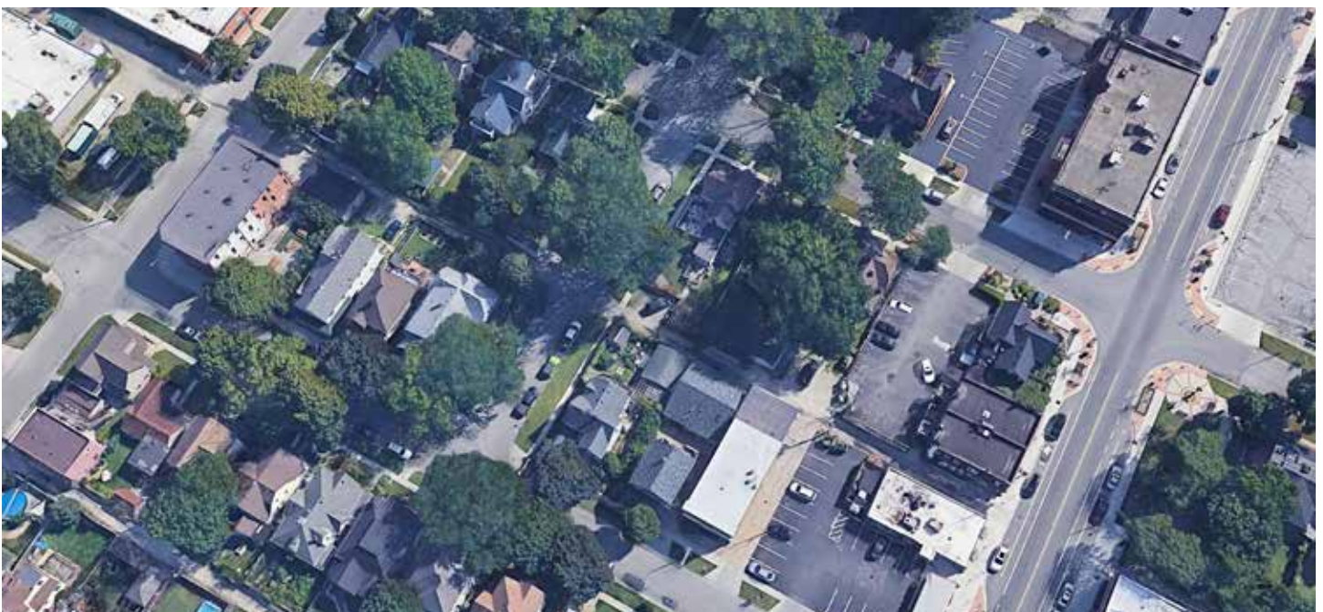
Bird's Eye View - Existing Condition
