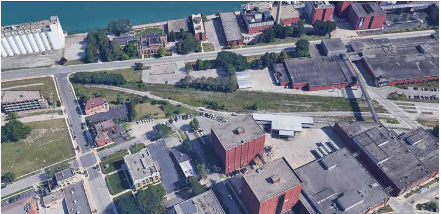
Bird's Eye View - Existing Condition
