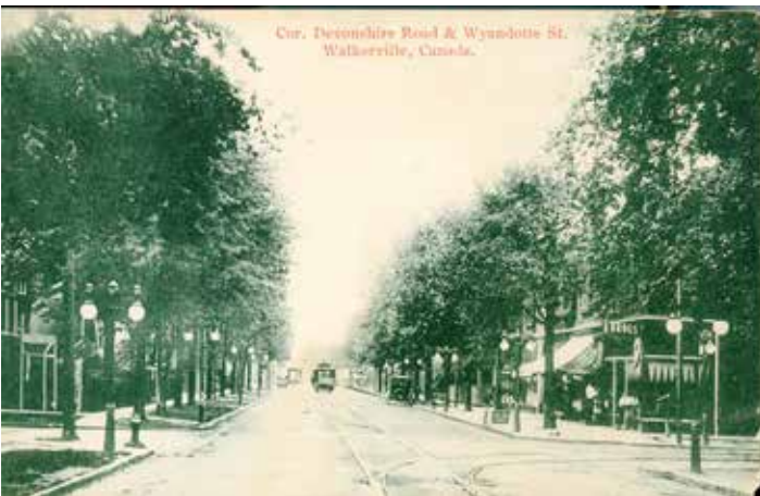
Image 1P: Corner of Devonshire St. at Wyandotte St. (1916) Image source: SWODA / Archives of Ontario
